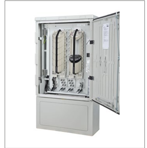
KVZ Street Cabinet with Single Fibre Management
