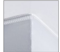
Clear Track Hallway Fibre Pathway
